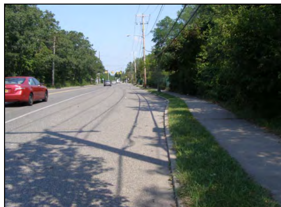
Picture 16: Excess Right of Way Station Rd
