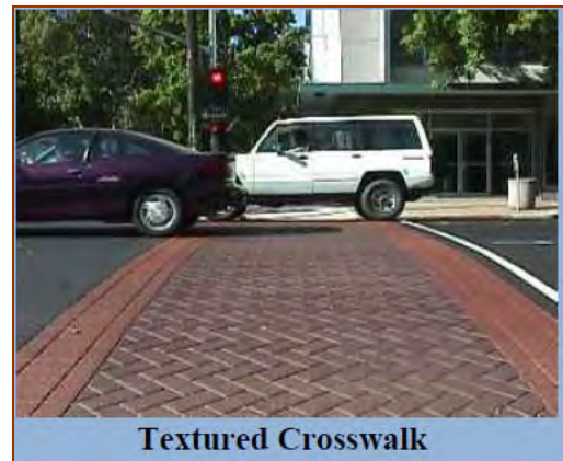
Picture 35: Textured Crosswalk
