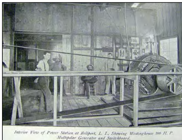
Picture 3: Monorail Power Station
