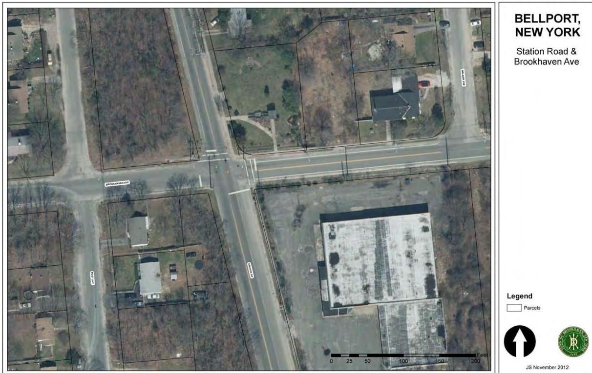
Figure 14: Intersection of Station Road and Brookhaven Avenue
