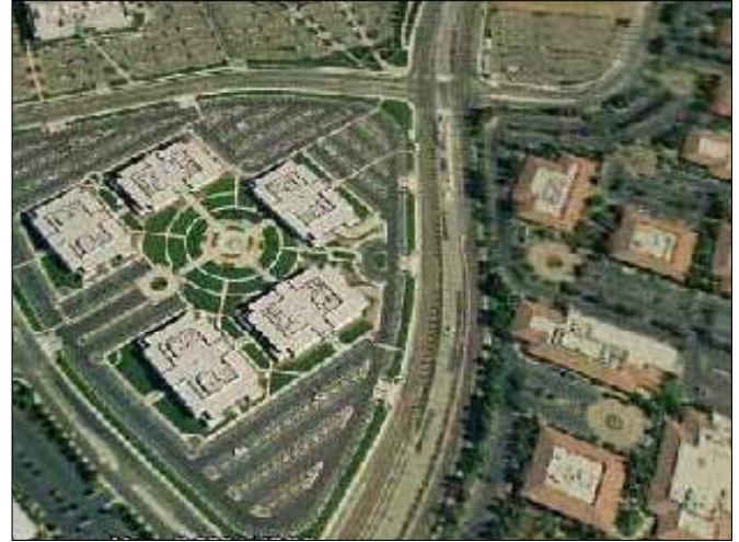
Acres of land is wasted on parking lots which could have been dedicated to park land, open space or workforce housing.
